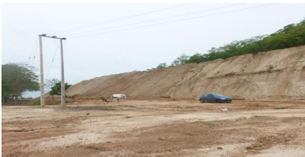
Plate 1: Massive earthwork at the road construction site on the Lokoja-Abuja highway.
