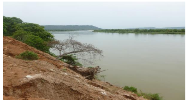
Plate 2: Deposition of tons of earthworks into the River Niger
